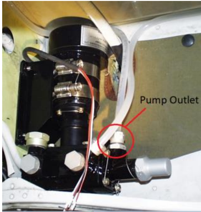
Figure 2: Pump Outlet Location
